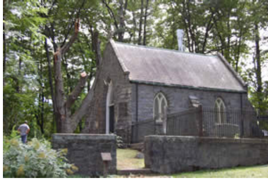
Durham's Smith Chapel was built in 1900 as a tribute to philanthropist Hamilton Smith. Modeled after the chapel in England where poet Alfred Lord Tennyson's father was rector, it is constructed in the English Gothic style with stone buttresses at each corner.
