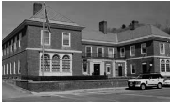
Peterborough Historical Society. One of the first purpose-built historical society buildings in New Hampshire, this museum was funded and designed by Benjamin Russell in the Georgian Revival style and built from 1916-1920. It continues to serve as both a historical organization and a multifaceted cultural organization for the Monadnock region.
