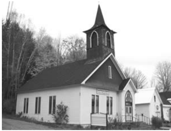
Stratford's Methodist-Episcopal Church , now the Marion Blodgett Museum, was the first church in town in 1853. In 1896, when a more modern building was desired, the frugal townspeople stripped the original building down to its frame, added a bell tower and vestibule, and created the shingle-style building that exists today. It was used as a church through the late 1950s and became property of the Cohos Historical Society in 2001.
