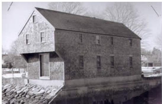
Sheafe Warehouse, Portsmouth. This warehouse was built circa 1720 using plank construction and was designed to make the loading and unloading of cargo boats, especially Piscataquag gundalows, as efficient as possible. Moved to Prescott Park in 1940 it is the sole survivor of a building type once common on Portsmouth's waterfront.
